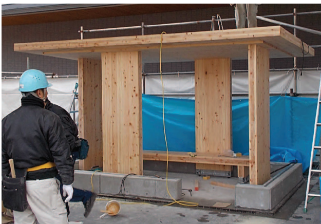
Bus shelter in front of Maniwa City Hall without drop walls or spandrel walls
