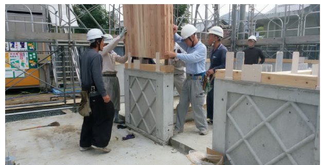
Installation of CLT panels. Connectors are left exposed and therefore coated for protection.
