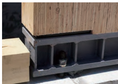
Metal Connectors/Fasteners for Wall Column
