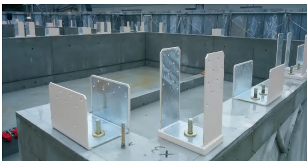
Shear connectors (left) and tensile connectors (center).
