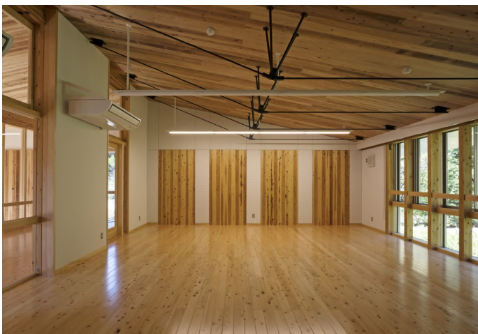
Kochi Prefectural University of Forestry with a roof structure using tension beams
